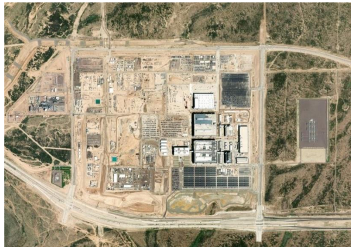
Aerial view of TSMC's facility under construction outside of Phoenix, Arizona. (Source: U.S. Geological Survey)
